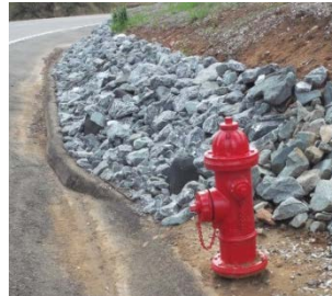
Crystal Swale Erosion Control
